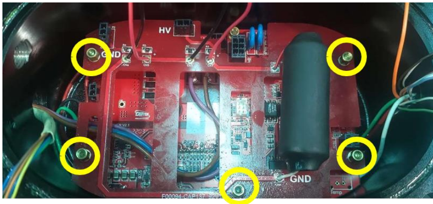
Figure 12 - Control Board Installation-9
