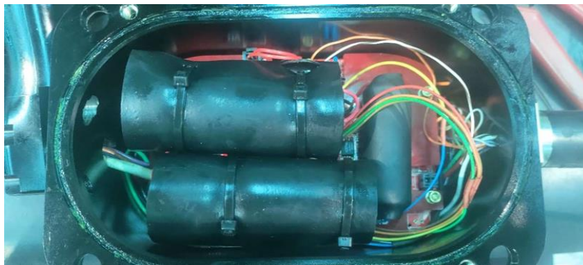
Figure 15 - Control Board Installation-12
