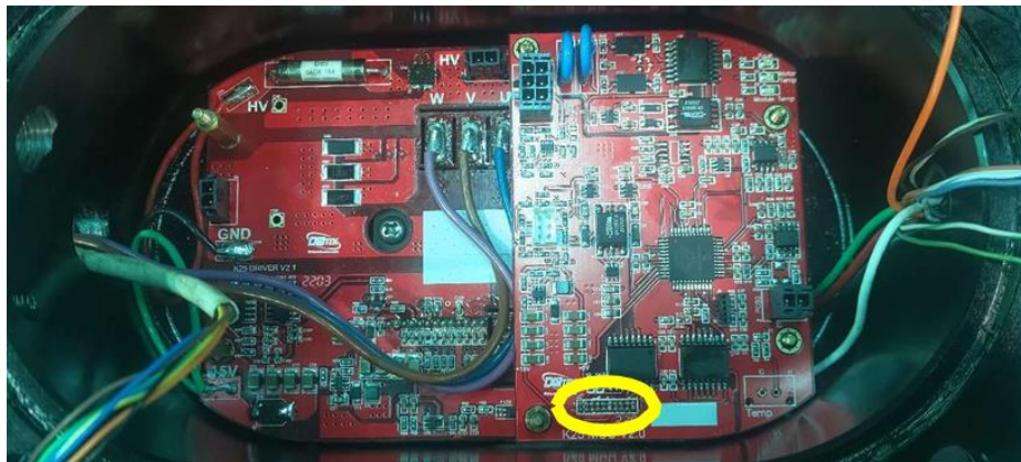
Figure 8 - Control Board Installation-5
