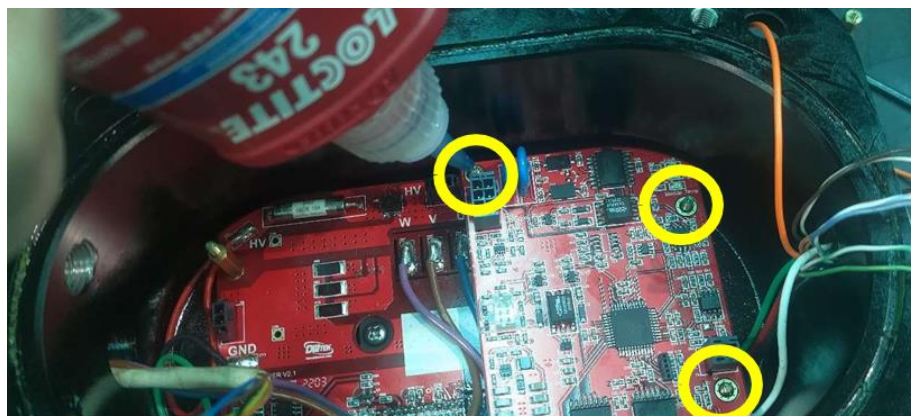
Figure 9 - Control Board Installation-6
