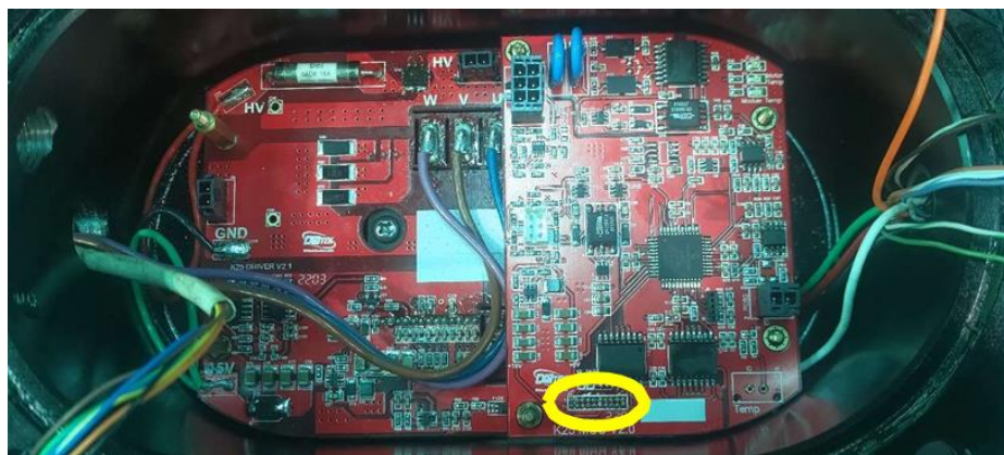
Figure 8 - Control Board Installation-5
