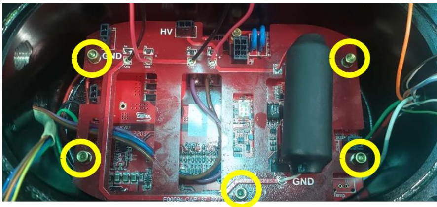
Figure 12 - Control Board Installation-9
