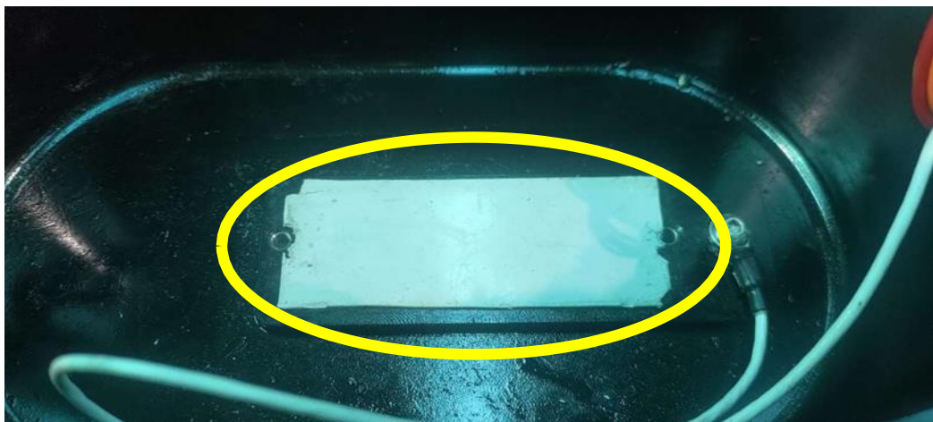
Figure 4 - Control Board Installation-1
