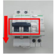
Figure 62 - AC Power Switch Off position diagram
